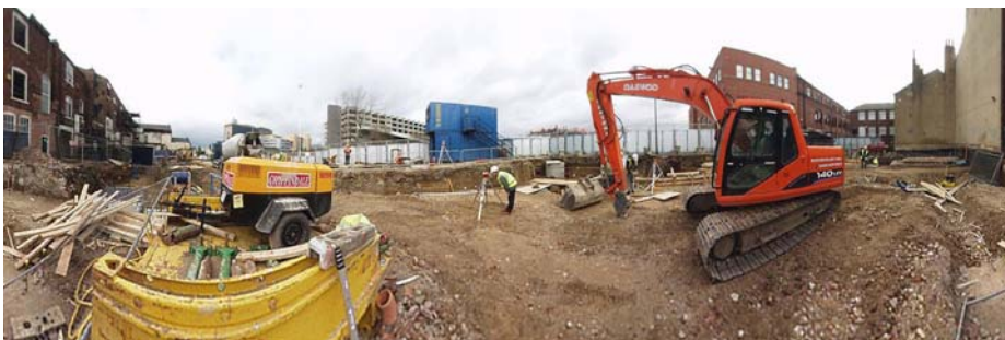
Figure 2c: 360 degree view of the construction site
