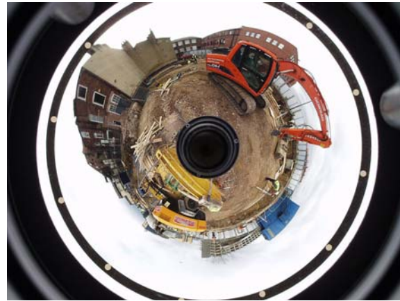
Figure 2 Donut shaped image of the site
