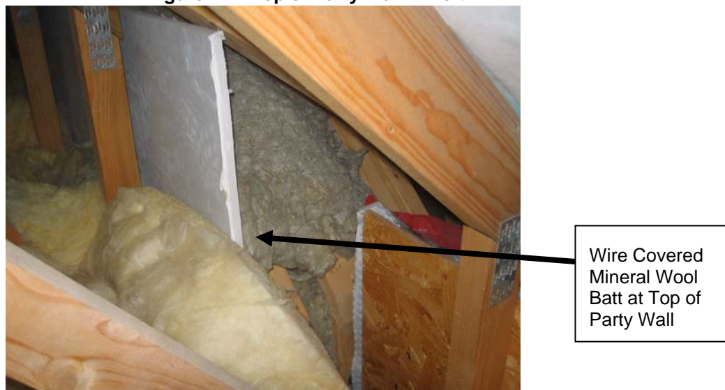
Figure 12 – Top of Party Wall in Loft
