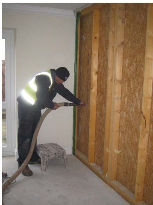
Figure 14 – Cavity Wall Technician Filling Party Wall at Darlington
