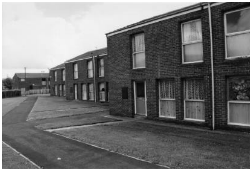
Figure 1.1 View of field trial dwellings before refurbishment
