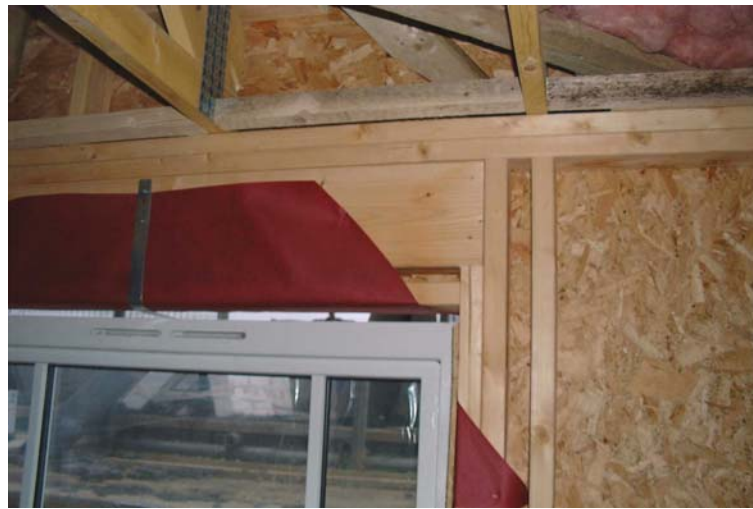
Figure 5 Typical window arrangement.
