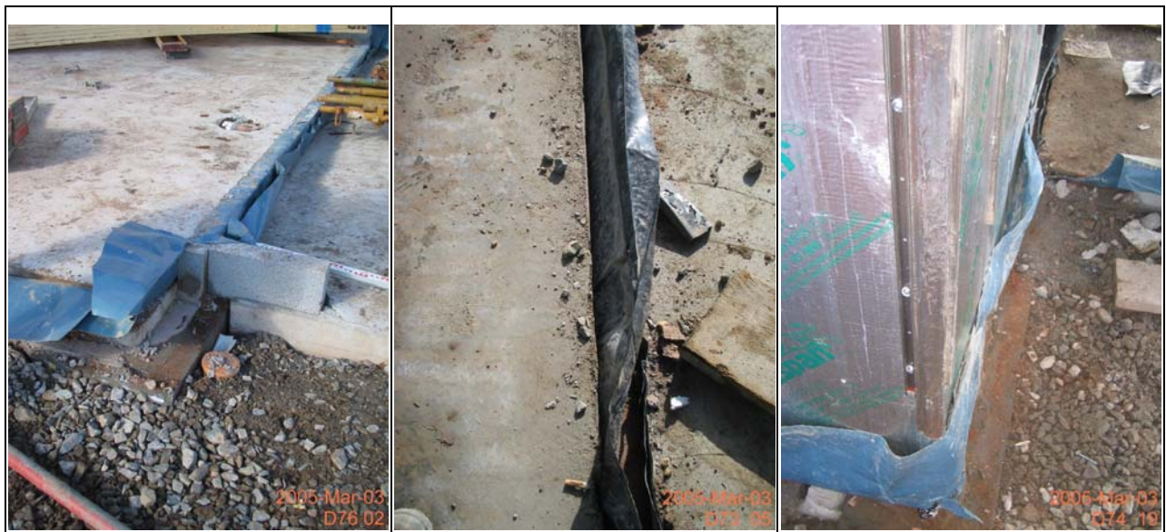
Figure 18 Developer D, Phase 3, using sacrificial blockwork to form the slab; after the blockwork is removed a straighter and more uniform slab edge reduces the potential for air leakage at this junction.
